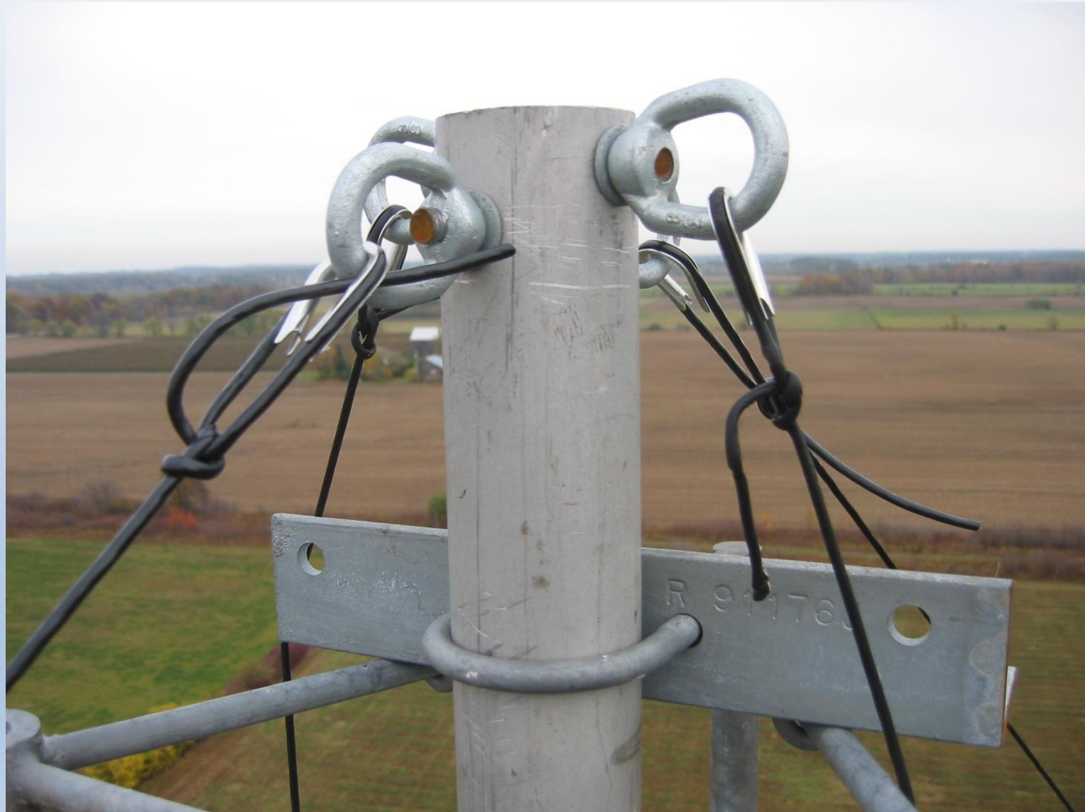
Catenary wire attachment at top of tower.
