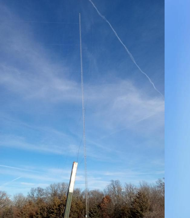
Ground mounted vertical element for 160m four square
