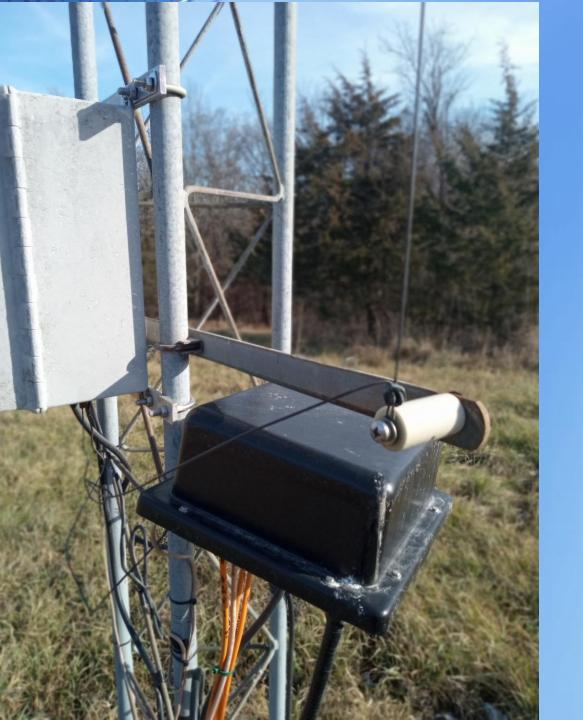
Bottom termination of tower detuning stub
