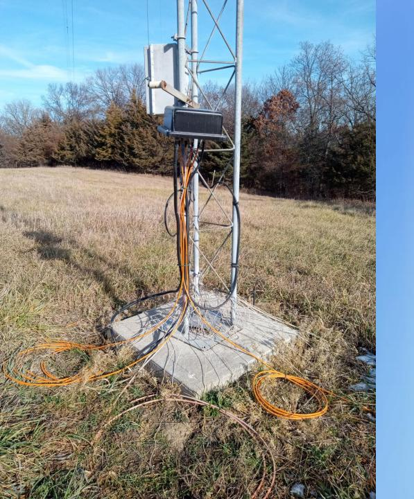
**Base of** 160m four square tower - 36 120' radials tower used only to support the four square vertrical elements
