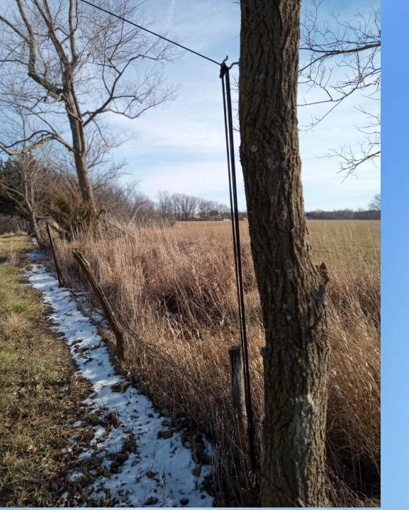
Securing the catenary rope supporting 160m vertical element
