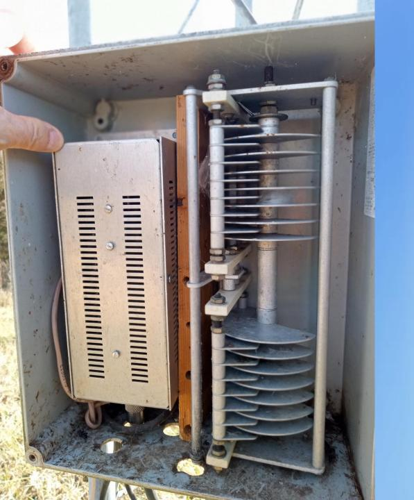
Dummy load for four square controller; cap for detuning stub – tuning stub currently disconnected
