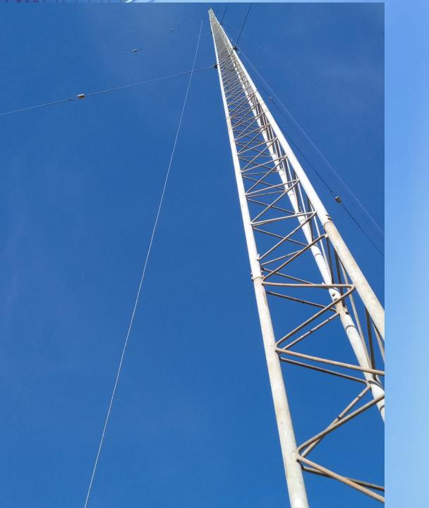
**Tower and** detuning stub **-12**" spacing; attaches to tower @ 100' levelterminates at 4' level with 87 pF cap to ground
