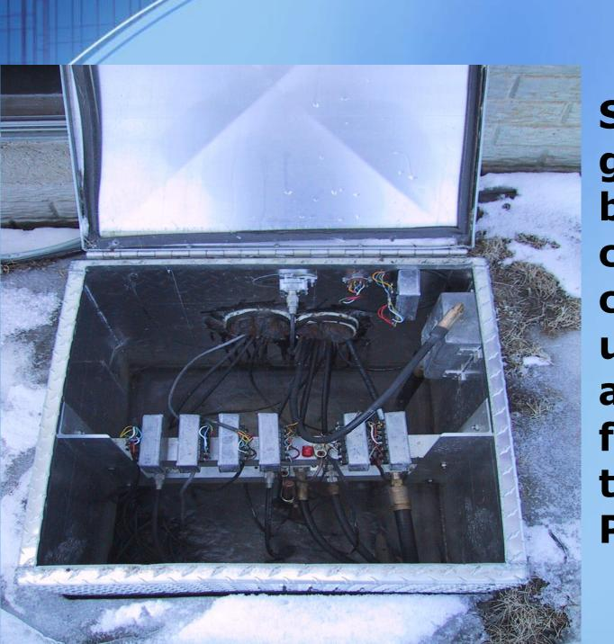
Single point grounding box -all cabling comes in underground and enters foundation through **Polyphasers**
